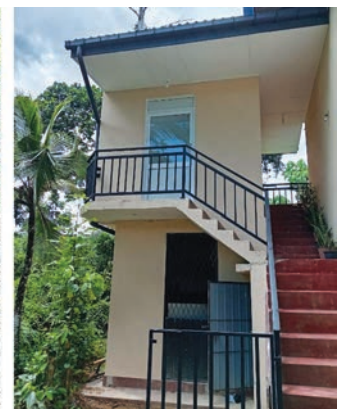
Construction of library building – Katandola welfare society
